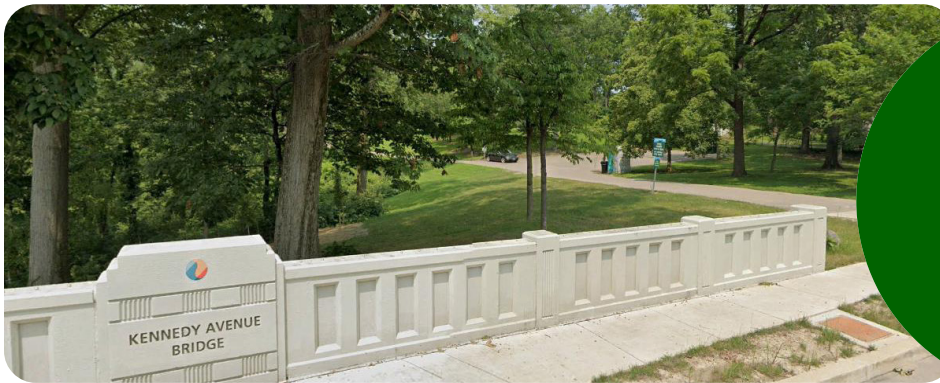
Kennedy Avenue Bridge & Kennedy Heights Park
